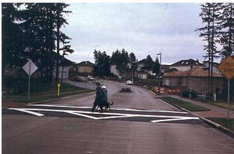
XV. Traffic Circle: Provides circular, counter-clockwise operations at intersections by placing an elevated area in the middle of the intersection. Approaching vehicles yield to traffic already in the circle. Street grades approaching the intersection shall not exceed ten percent.
